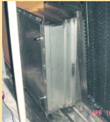
Here you can see the depth of the 'hobbit' door access hatch.
