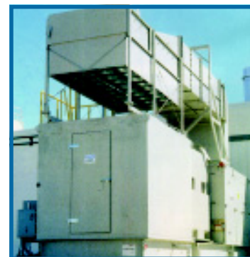
TTD self-cleaning air filter protects a Solar turbine in the hot, arid, dusty environment in Nevada USA.
